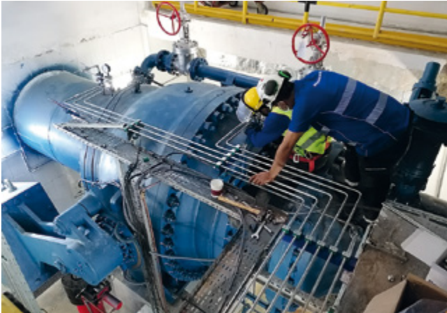
- Installation of hydraulic systems worldwide
